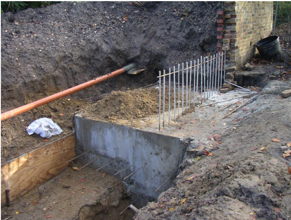
Photograph 6: Boundary wall repairs
