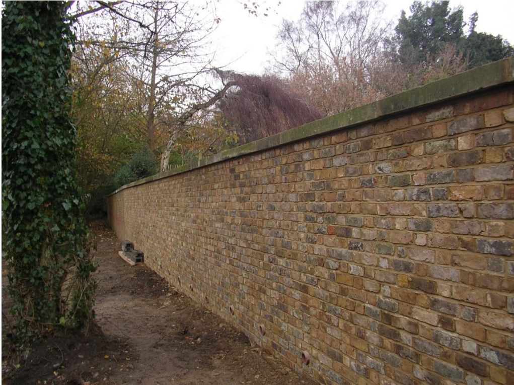
Photograph 7: Completed boundary wall repairs
